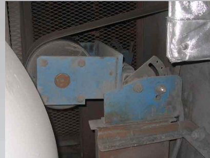
Side view of the Lovejoy ROSTA Heavy Duty Tensioner
